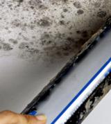
Corrosion of sprinklers, fittings, pipe, hangers and components
