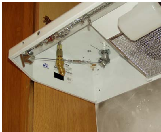
Figure 2-2. One side of a “typical” wet chemical system; two thermal links and a nozzle are shown, the opposing side was similarly configured.
