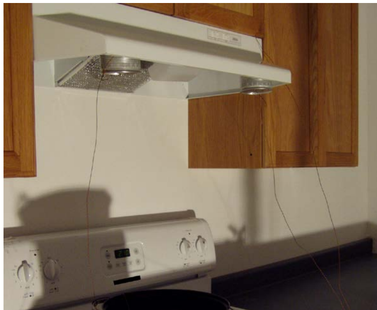
Figure 2-5. Autonomous dry chemical system installed above the stovetop. The thermocouples seen in the image were added and were not an intrinsic part of the device.
