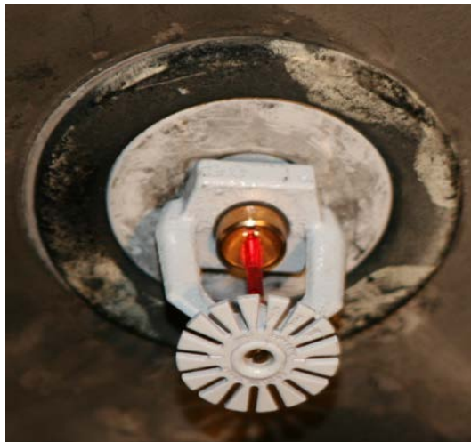
Figure 2-7. Water sprinkler head.
