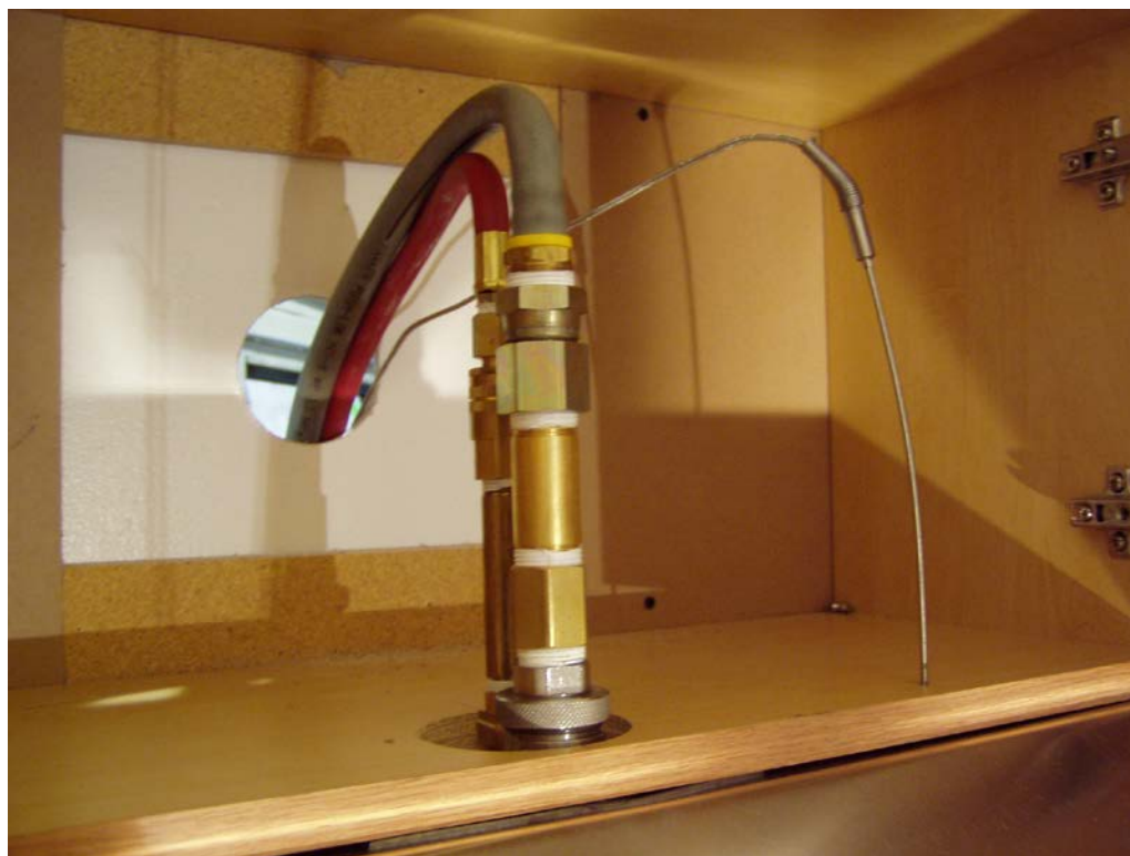
Figure 2-6. Plumbing for a water mist system above the range exhaust hood.
