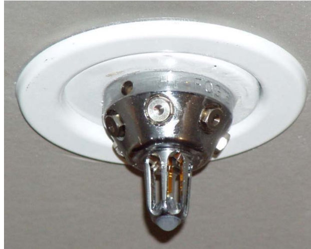
Figure 2-8. Water mist nozzle.
