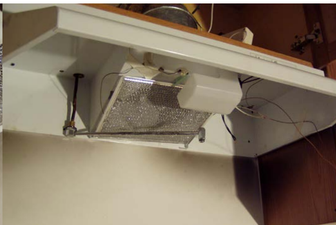
Figure 2-3. AWC3 was a single nozzle system that used an electrical thermal trigger.
