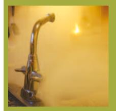
The system uses a high-pressure pump to generate a fine water mist from nozzles mounted under a kitchen monobloc tap, on a work surface or in a wall. Versions are available for protecting living rooms, kitchens, and open or semi-open kitchen/diners.
