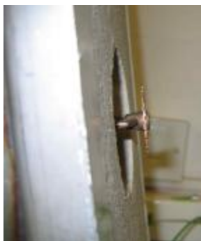
Concealed head installed at maximum recess distance prior to attachment of concealer plate
