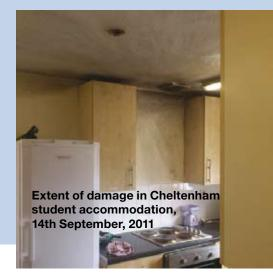
been fitted with sprinklers. The fire was extinguished by the actuation of just a single sprinkler head and damage was confined to light smoke damage and water on the floor. The accompanying photograph testifies to the effectiveness of the sprinkler system.
