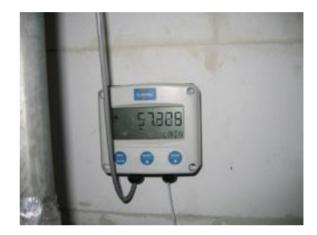
Sprinkler flow-rate meter
