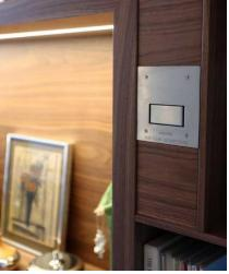
Figure 20: Preferred position built into a cupboard or joinery
