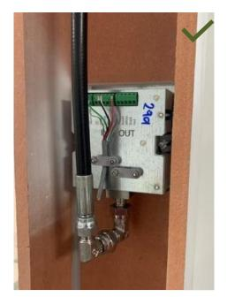
Figure 53: Correct trunking installation with double elbows
