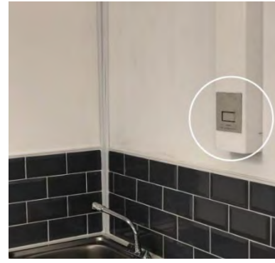
Figure 33: Preferred position behind a sink
