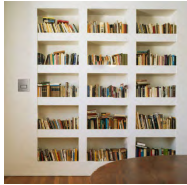
Figure 32: Preferred position alongside a recessed shelf
