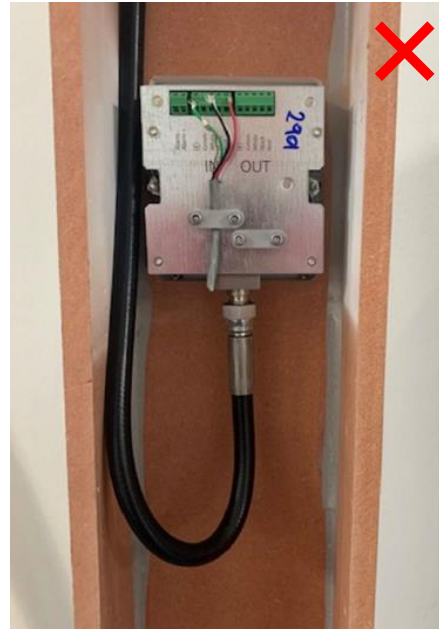
Figure 54: At risk trunking installation with hose bending
