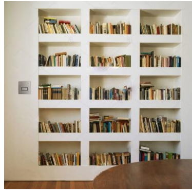
Figure 32: Preferred position alongside a recessed shelf
