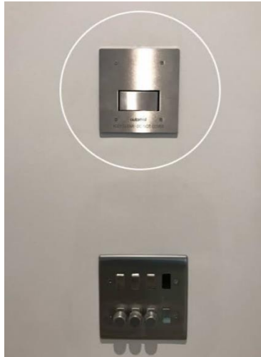
Figure 19: Preferred position within 30cm of a light switch
