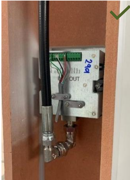
Figure 53: Correct trunking installation with double elbows
