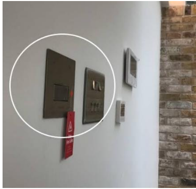
Figure 31: Preferred position alongside a light switch
