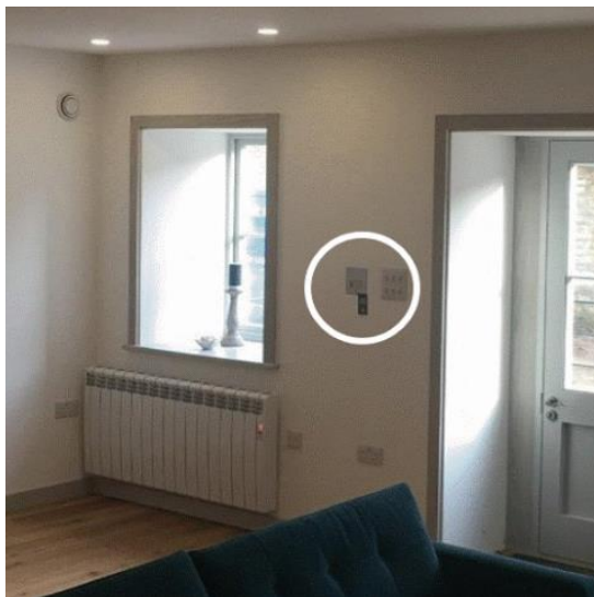
Figure 29: Preferred position alongside a window
