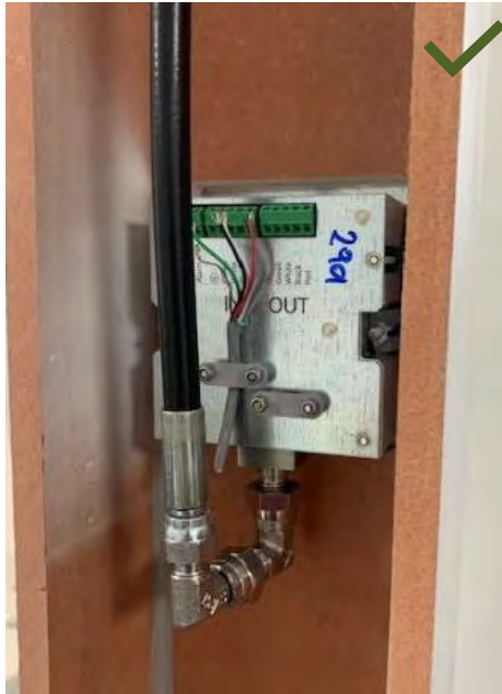
Figure 53: Correct trunking installation with double elbows
