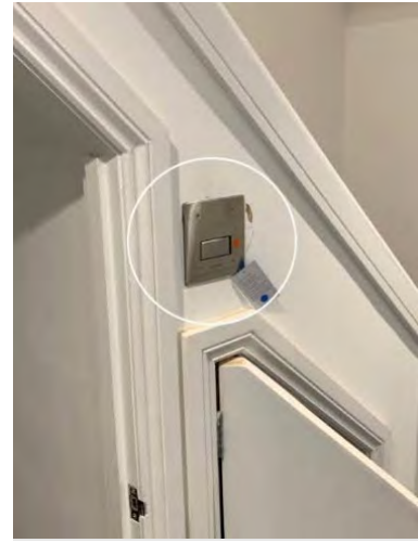
Figure 21: Preferred position on a staircase
