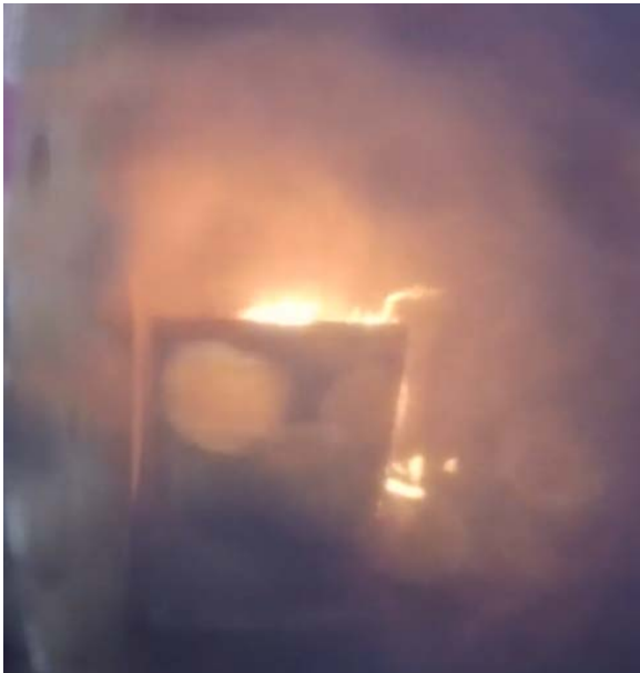
Photograph of system during test 1
