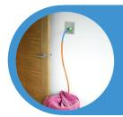
Your installer will test the system to ensure that it is working correctly. Piping will be used to safely direct spray into a bucket.
