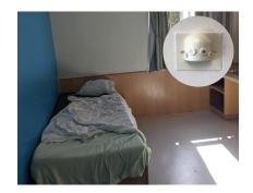
A custom pre-engineered Automist fixed system was the ideal solution for 14 rooms in Prospect Park Mental Health Hospital. It featured an antiligature head and a key switch control outside each room which staff could operate. The installation was completed in one day to minimise patient disruption.
