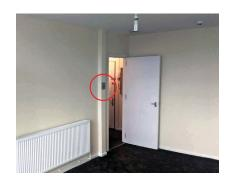
Automist has been installed in 11 sheltered housing schemes in Lambeth. As the system connects to the existing water supply, it is often more cost effective to retrofit than sprinklers and can be fitted quickly, minimising disruption to residents and the fabric of the building. Automist can be fitted on a flat-by-flat basis, so protection can be targeted to the most vulnerable first.
